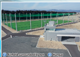
7 Airfield surrounded by net 2 Hangar
