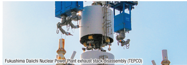
Fukushima Daiichi Nuclear Power Plant exhaust stack disassembly (TEPCO)
