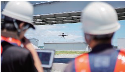
Drone flight under test bridge girders
