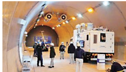
Detection of internal tunnel defects using cameras, radar and lasers
